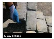
Lay patio stones in the desired pattern. If the desired pattern requires cutting, the patio stones can be cut with a wet saw.
