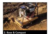
Install patio base to a compacted finished thickness of 4 in. (102mm) for patios and walkways.
