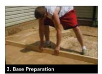
Lay a 1 in. outside diameter pipe on base. Spread 1 in. of sand over compacted base. Level the sand by dragging a 2 in. x 4 in. (51mm x 102mm) board over pipe.
