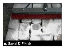
Spread polymeric sand on the installation and sweep into joints, according to manufacturer's instructions. Sweep off any loose sand from project surface.
