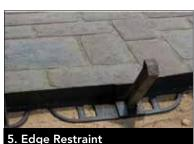
Install paver restraint edging and spikes around the entire project, according to the manufacturer's instruction.
