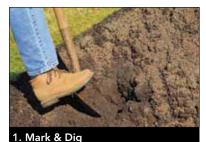
Excavate the installation area to approximately 6 in. (152mm) larger on all sides than the actual finished size.
