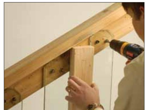
**Step 1:** Attach top and bottom stair rails to posts according to local building codes. The distance from the front edge of the stair tread to the top of the rail is typically 36". Use a baluster as a guide to determine placement of the bottom rail. Find the center of the top and bottom rails and mark.
