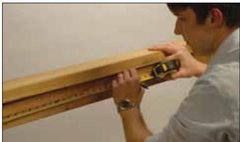
**Step 1:** Attach top and bottom rails to posts according to local building codes. The distance from the deck surface to the top of the rail is typically 36". Use a baluster as a guide to determine placement of the bottom rail. Find the center of the top and bottom rails and mark.
