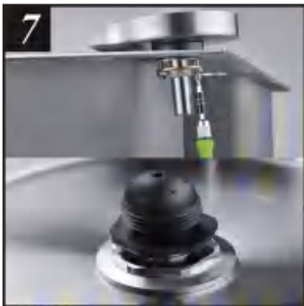
7. Thread the 1/2" end of provided supply line to mounting shank with wrench.
