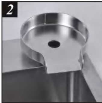
2. Put the base on the sink hole
