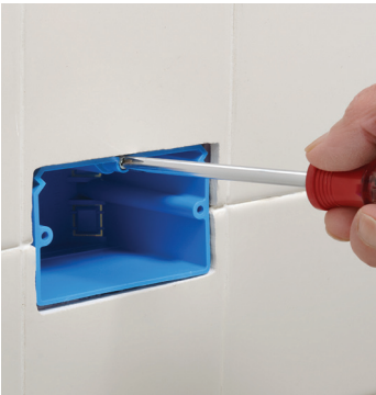
Turn the Adjust-A-Box® screw after installation to bring the box flush with the wall surface.
