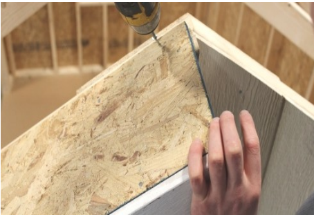
(134) Fasten the top as shown.
