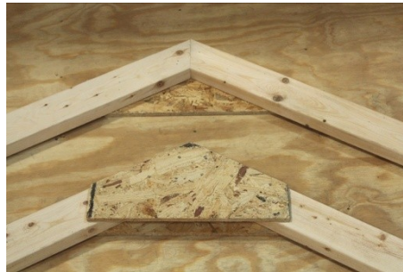
(117) Lay out the rafter pieces and the gussets. Note: Two rafters will be assembled using only one rafter gusset, the remaining rafters will be assembled using two rafter gussets.
