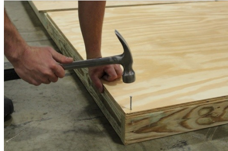
(24) Attach the corner of the flooring, using 2" nails.
