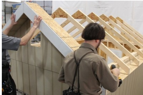
(135) Install right gable overhang, repeating previous steps.
