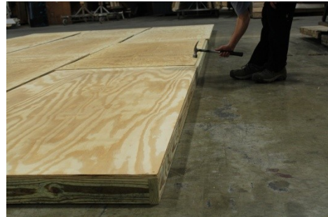
(26) Nail along the front side, making sure flooring is flush with the band board.
