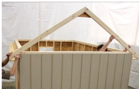
(120) Begin with end rafter keeping single gusset facing to interior of shed as shown.
