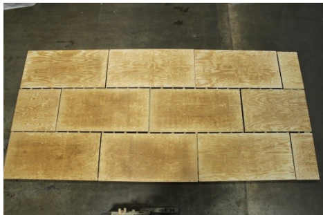
(22) Layout the flooring as shown.
