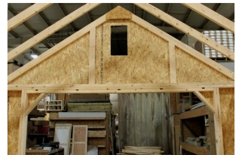
(142) Fasten the other gable brace on this gable, then repeat for opposite gable. Next, fasten the siding splices to the gable braces on the outside.
