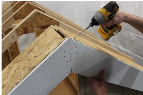
(137) Correct! Fasten firmly, using a 3" screw.
