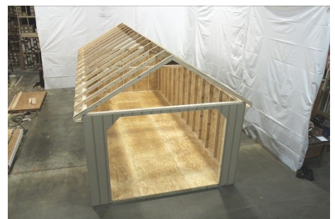
(124) Install the rest of the rafters, 24" on center, or in every dado groove on the top plate. Repeat, till all rafters are installed.
