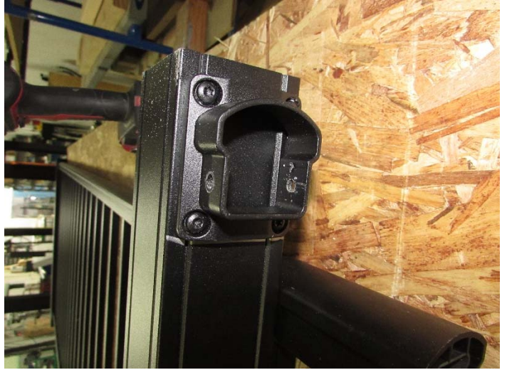
Top Bracket Profile Detail
