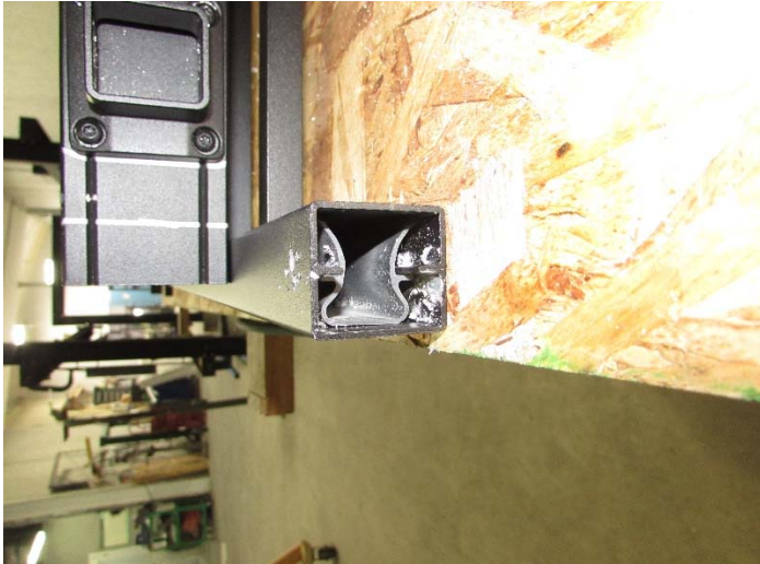
Bottom Rail Profile Detail
