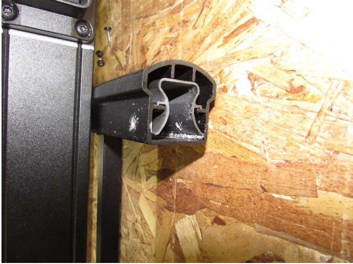
Top Rail Profile Detail
