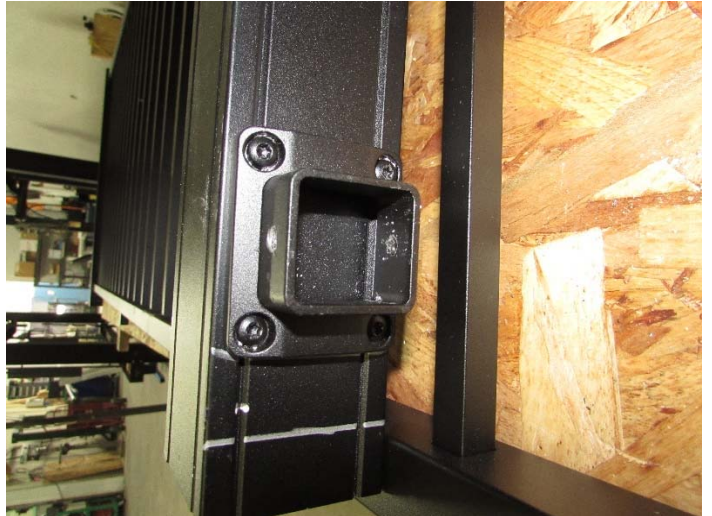
Bottom Bracket Profile Detail
