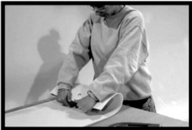
**USE 'M77' SLIDE BRACE AS A TEMPLATE FOR DRILLING BOTTOM HOLE PATTERN IN SLIDE BED. BE SURE TO PLACE SLIDE BRACE UP 1/4" FROM BOTTOM EDGE OF SLIDE BED BEFORE MARKING HOLE PATTERN.**
