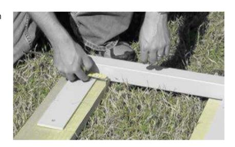
Then using a 3/8" drill bit and the INSIDE hole as a guide (closest to the frame), drill through the planks for the inside hole on each plank and secure with a 3/8" bolt, washer and nuts on each one before drilling the next. The carriage head should be on the outside face of the gate with the washer and nut facing you as you complete the gate frame.
