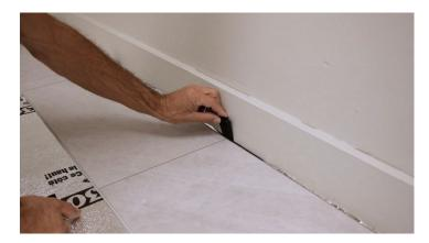
The end joints of the planks in the first row are assembled by overlapping the tongue side over the groove side of the previous plank ensuring that the planks are perfectly aligned, with firm pressure; push the end joint downward till the end of the plank snaps in place. Install remaining full planks in the first row
