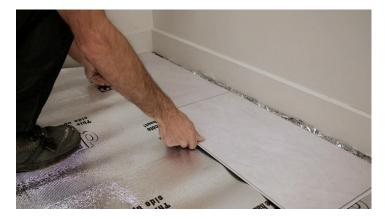
Place 3/8" (9.5mm) spacers between the short and long side of the planks and the wall. Always position one spacer between the wall and where the planks join.
