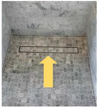
Linear drains simply require pitching the floor towards the drain site. Allowing for placement options not limited to the center of the shower, curbless designs and easier installation with all flooring options including large format tiles.
