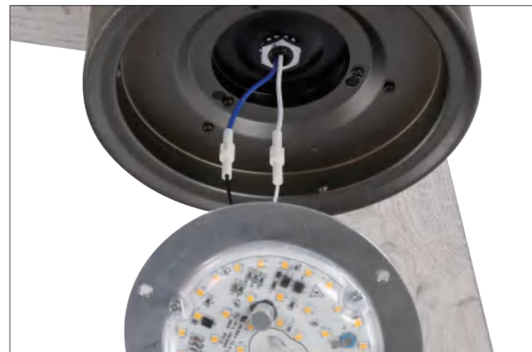
Step 11 Connect the wires of the light source.
