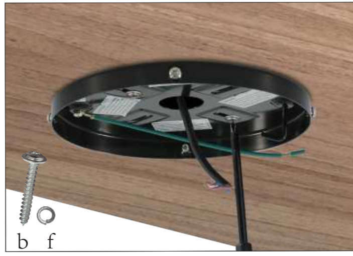
Step 1 For wooden ceiling, install the mounting plate to wooden ceiling with two wood screws.
