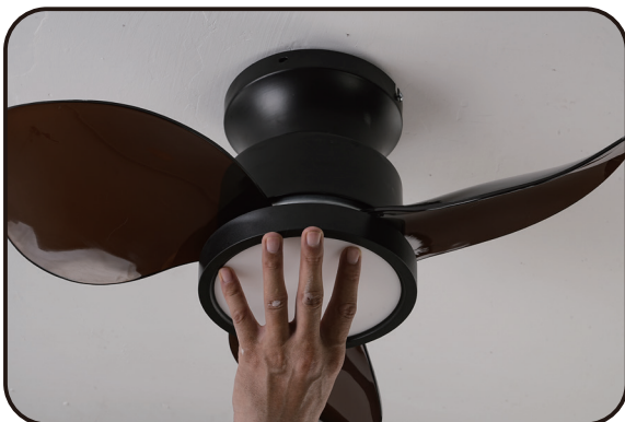
Step 9: Hang the whole ceiling fan to the ceiling mounting base.
