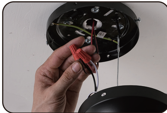
Step 8: Connect the AC cables and ground wire.
