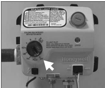
Figure 43: Gas control/valve.
