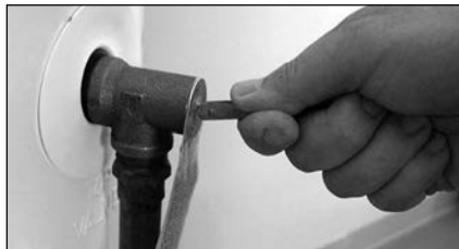
Figure 41: T&P Relief Valve.
