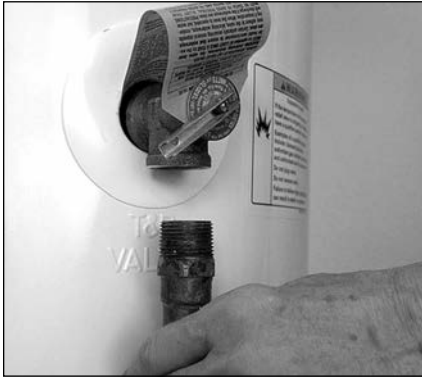
Figure 13: Removing the T&P Relief Valve discharge pipe.
