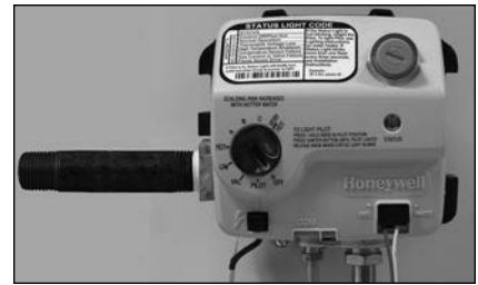
Figure 47: Gas control/valve with threaded pipe.
