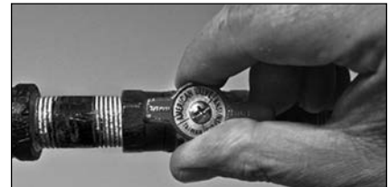
Figure 48: Gas valve in "on" position.
