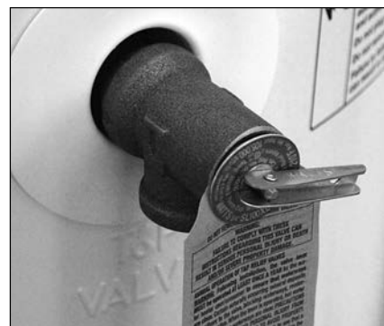
Figure 18: Temperature and Pressure Relief Valve
