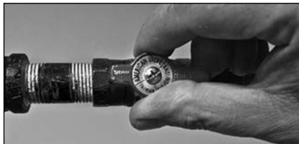
Figure 30: Gas valve in "on" position
