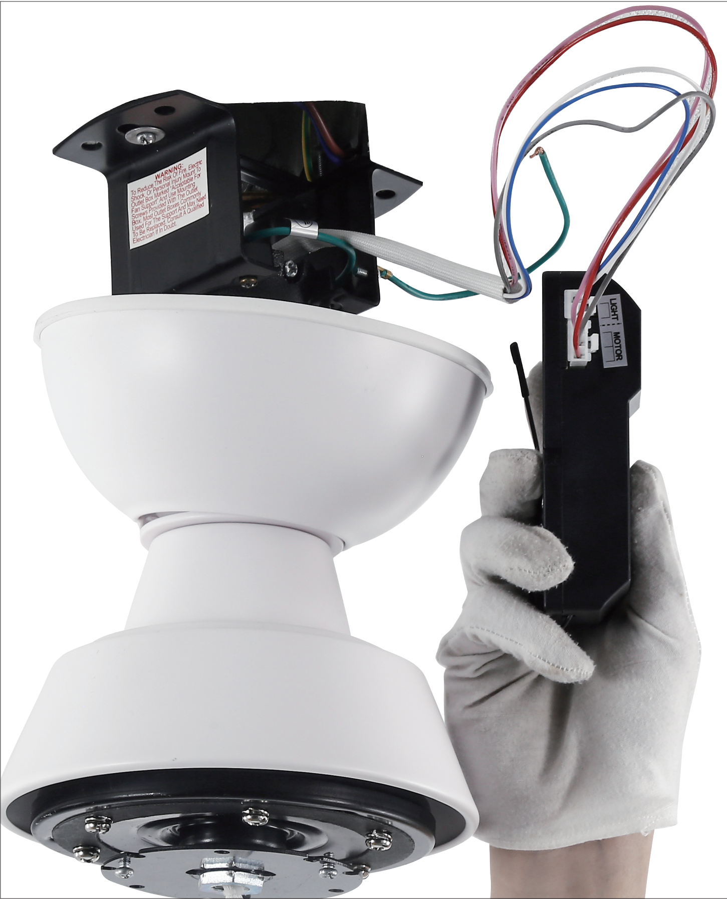
Step 12 Connect the wires from motor to receiver.
