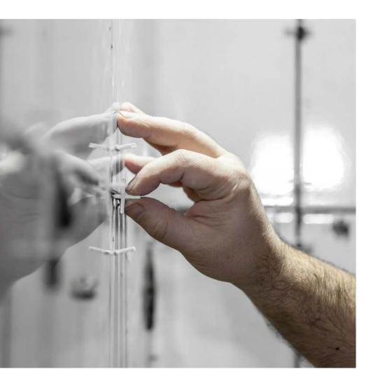
Joints must always be left between the tiles to guarantee the surface's proper technical performance.
