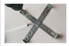
1. The hanging board is fixed on the ceiling with screws
