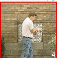
Mix the mortar according to the instructions on the bag. Apply the mortar around the perimeter using a grout bag or a trowel. Make sure the joints are completely full.
