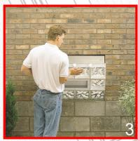
Set the new window into place on top of 2 wood wedges, check that it is plumb and level, then secure it with 2 wood wedges at the top. If you are installing a vented window the vent latch should be located on the inside at the top.
