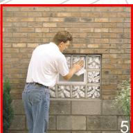
When the mortar begins to set, remove the wedges, fill the holes, smooth the joints with a trowel and clean the glass with a clean cloth.
