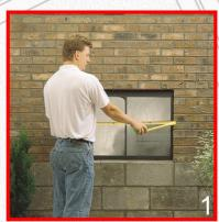
To make sure your new window will fit properly, the measure window opening as if the frame were already removed. You will need a space of approximately 1/4" to 1" all the way around the perimeter for mortar.
