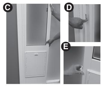
Step 3: Now that the Pet Patio Door Panel is in place, attach the Filler Insert (F) into the top spring section opening and press into place Note: if you need to remove the Pet Patio Door Panel, be sure to remove the Filler Insert first.
