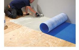
Spread only as much mortar as can be covered with Mapeguard UM 35 [NA] before the mortar skins over.
