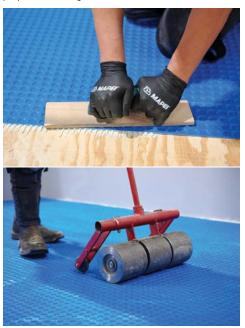
8. While laying the rolls of the membrane, it is recommended to leave a 3- to 5-mm gap between the sheets. To ensure a flat surface, do not overlap edges or ends from one roll onto another. Leave about 1/4" (6 mm) between the membrane and the edge of walls, columns, etc., for movement.
