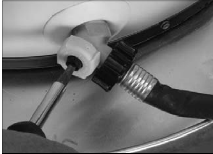
Draining the old water heater.
