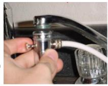
diverter valve lever to the left slowly so that its perpendicular to the spout. Water will flow through system and dispense from smaller outlet on the diverter valve. Some water discoloration and air bubbles may be present due to loose carbon. Allow water to run through system for 5 minutes until water runs clear and free from air bubbles.
