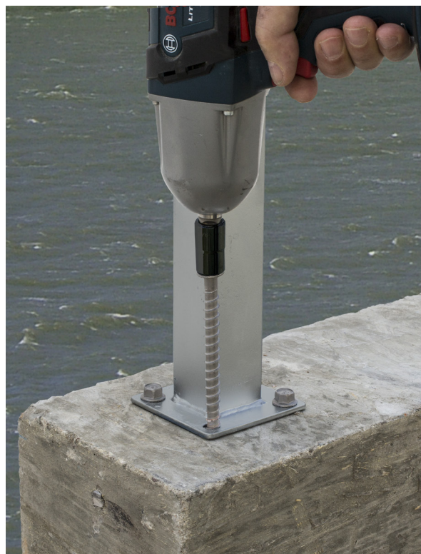
Installation of stainless-steel Titen HD screw anchor.
