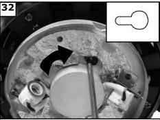
Lift light kit to the fan motor assembly. Align the 3 screws with the key hole slot holes in the light kit (see inset). Rotate the light kit as shown. Then install the screw removed in the previous step though the closed hole. Tighten all 3 screws securely.
