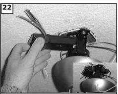
Install remote receiver by sliding into opening in the Mounting bracket. Make sure that the dip switches on the Transmitter and the Receiver are set to the same position. See Fig 39 for remote operation
