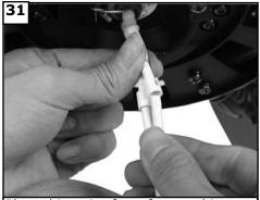
Plug white wire from fan to white wire from light kit. Then plug black wire from fan to black wire from light kit.
