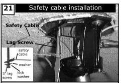
Fan and light kit combinations over 35 lbs, in both flush and downrod mode the safety cable must be installed into the house structure beams using the 3" lag screws,washers, and lock washers. provided. Make sure that when the safety cable is fully extended the lead wires are longer than the cable and no stress is placed on the lead wires.
