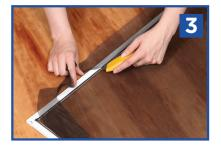
3. Trim off excess screen with utility knife on outside edge of the spline groove.
