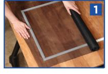
Lay screen over frame on flat surface, overlapping spline groove at least 2" on all four sides.
