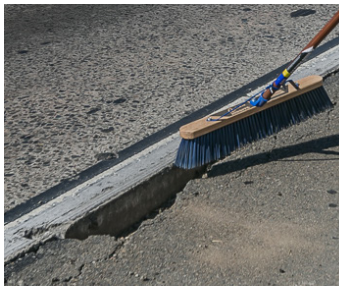
Clean Repair Area
