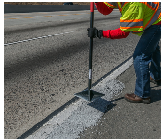
Tamp Repair Area
