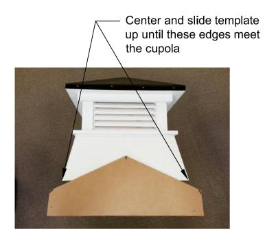
**6.**Once template is centered and in place, trace lines onto the cupola.
