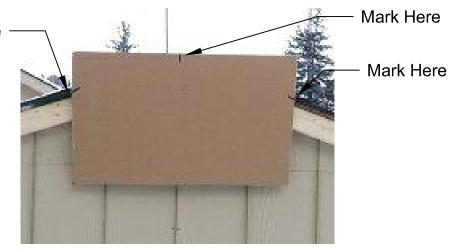
Center two rafters flush to the top of the template.
