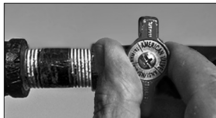
Figure 43 - Gas shut-off valve in "off" position.
