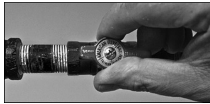
Figure 32 - Gas valve in "on" position
