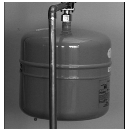
Figure 14 - A Thermal Expansion Tank helps protect the home's plumbing system from pressure spikes.
