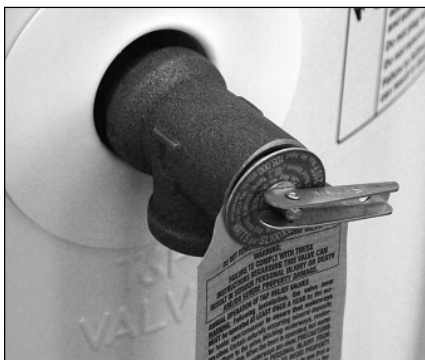
Figure 25 - Temperature and Pressure Relief Valve
