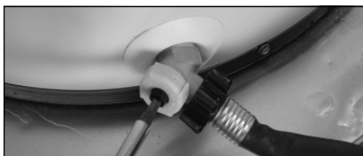
Figure 37 - Draining the water heater.
