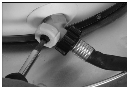
Figure 21 - Draining the old water heater.
