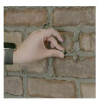
7. As you use the jointer, if you come across a spot that doesn't have enough mortar, pick up some of the excess that has just fallen away from the section you are working and push it into the gap. This ensures that the mortar you add has the same level of dryness as the surrounding material.
