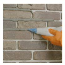
4. Hold the grout bag with one hand in the middle and one hand at the end where it is twisted. Put the tip of the bag in the space between the bricks at a 45 degree angle. Twist the end of the bag and squeeze as you move the tip along the gap. The grout should over fill the gap just a little so that you have enough to tool later. This process takes some practice. \*Do not try to wipe off excess while the grout is wet.\*
