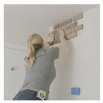
4. Apply your first sheet of Brickwebb in a top corner and then move horizontally. Press firmly on the bricks so that the adhesive comes through the webbing and adheres. Check that your section is level and make adjustments as needed while the adhesive is still wet.
