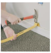
3. Then use a pry bar and a hammer to pull the baseboard from the wall. Be gentle and do this a few times before pulling the full baseboard off so that you don't damage the wall.
