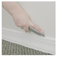
2. Remove any baseboards and trim that are less than 1/2" thick. To remove a baseboard, start by scoring the caulk with a box cutter or other sharp knife.
