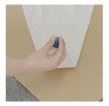
2. Trim the end of your grout bag so that the opening is about ½" wide. Then fill your grout bag by folding down the top edge of the bag and then step on the tip of the bag. Use a trowel to fill the bag about half-way.
