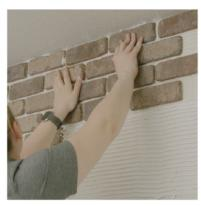
5. Apply your next sheet overlapping the first sheet, leaving %" between the bricks for grout. Repeat this process as needed.
