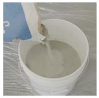
1. Mix the Type S mortar mix following the steps on the packaging.
