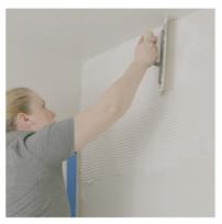
3. Use a notched trowel to apply the adhesive. Smear on the adhesive generously with the flat side first and then use the notched side to scrape off excess.
