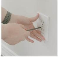
1. Remove any outlet covers, thermostats, and other items from the wall. Use painters tape to tape anything that you can't remove such as vents and adjacent walls.
