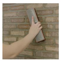
8. After the grout has had some time to dry, come back and brush away any excess left on your project. Using a stiff bristle brush, start with a small section and brush the bricks with a 45 degree angle stroke. If the mortar leaves streaks on the brick faces or leaves mortar on your brush, it is still too wet and you will need to give it more time to dry.
