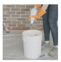
3. Unfold the top of the bag and hold it over your bucket of grout. Shake the back to remove bubbles and then twist until the grout starts to come out of the tip. The grout should come out when squeezed, but not be so runny that it drips out on its own.
