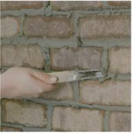
6. Use the heal edge of your jointer to push the mortar into the gap and away from you. The excess mortar should fall away and not stick to the brick face. If the mortar is sticking, it is still too wet and needs to set for a few more minutes. You should get clean edges with a slight indent in the grout.
