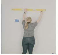
2. Starting from the top of the wall, measure down at 21" increments. Mark horizontal lines on the wall using a level. Apply adhesive and thin brick section by section.
