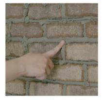
5. Start at the top of your wall. Fill in sections of about 4 square feet at a time. Give each section about 15 minutes to dry. You can do about 4 sections one after the other before going back with your brick jointer. When the grout is dry enough to touch without sticking to your finger, it is ready to start tooling. It should still be soft enough to squish a little.
