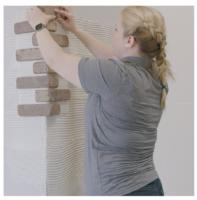
1. If your project includes corners, install your corner pieces first starting at the top of the wall using the following steps. After the corner sheets are installed use these same steps again to install flat sheets.
