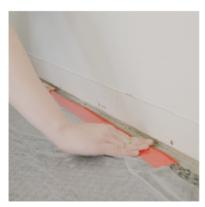
4. Put down some plastic covering on the floor and secure it in place with tape to protect your floors and for easy cleanup later.
