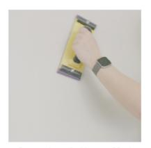
5. Go over the wall with some 80 grit sandpaper. Use a small circle motion and go over the entire surface of the wall. You don't need to push hard, the goal is simply to rough up the surface so that your adhesive improve bond.
