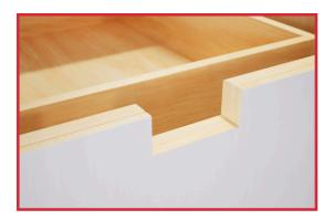
1. Mark 2"-4" from the outer edge of your cabinet for your first notch to be cut. Then set marks for the remaining brackets every 16"-20" apart. Rout or chisel out a 1" deep by 2.5" wide notch from the cabinet. Top of brackets should be flush with top of the cabinet.
