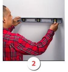
Use a level and tape measure to mark bracket locations.
