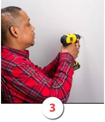
Pre-drill holes and insert screws with drill or screwdriver.
