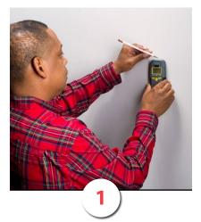
Plan shelf placement. Locate and mark wall studs using a pencil.
