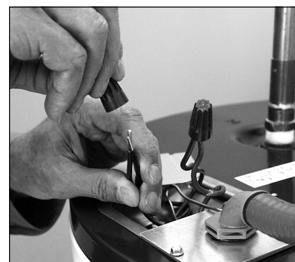
Figure 19 - Connecting the electrical wires.
