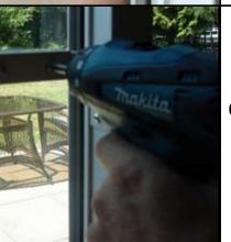
**06.** Make sure the Patio Door Bar is closed and in the fully extended position, drill the 1/2" self-tapping screws through the exposed Positioning Holes and into Positioning Channel. (Pre drill with 1/8" drill bit if necessary)
