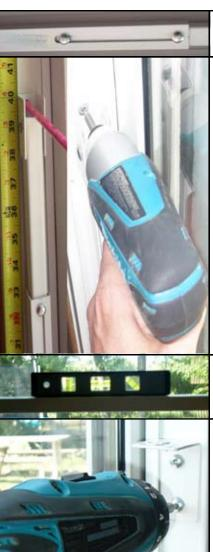
**01.** Fully extend Patio Door Bar and insert Carriage Bolt into threaded hole in slot.
