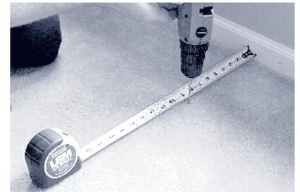
**Step 4.** Shift the drill into reverse. If the screw doesn't back out, the threads of the screw aren't in the joist. Lift the drill while you slowly reverse the drill, this will back the screw out. Move over an inch, moving away from the wall or the vent if you are using that, and drive it down again.
