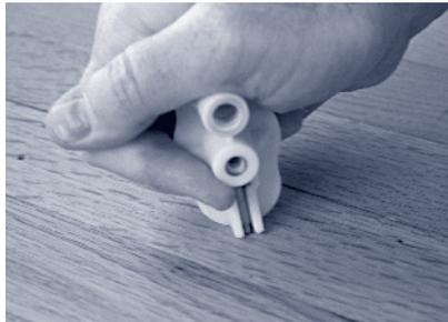
Rock the fixture or pliers back and forth until the head of the screw snaps at the score.
