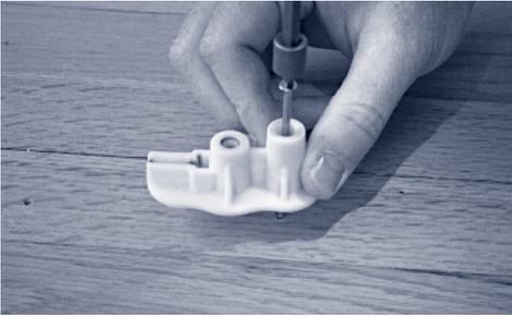
After pre-drilling a  $\frac{1}{8}$  inch hole down 2  $\frac{1}{4}$  inches, drive a screw through the taller opening in the fixture.
