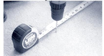
**Step 5.** Continue these steps until the screw comes up on its own indicating that you have gone into the joist. At this point you can measure across the room to the other joists. Floor joist are normally set on 16 inch centers.
