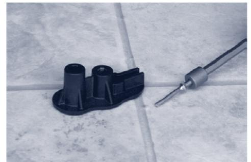
The screw is now set  $\frac{1}{5}$  of an inch below the floor. Take a hammer and tap the small bump that is left to smooth out the hole and force the hole to fill over.
