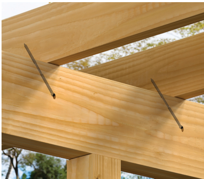
Joist-to-Beam Connections
