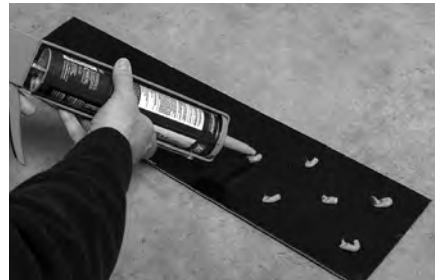
Method 2 - Using high-quality polyurethane construction adhesive
