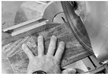
Chop saw can be a cutting option for straight cuts
