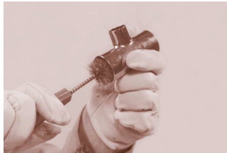
Figure 5. Cleaning: Fitting Brush
