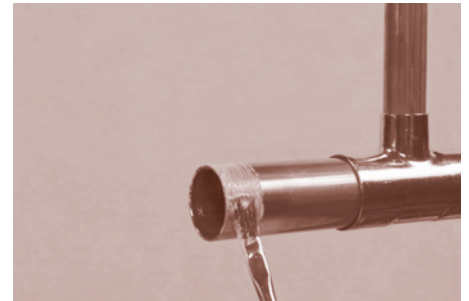
Figure 6. Fluxing: Tube
