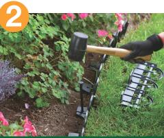
Hammer spikes through tabs at the ends of the installation and connection points. Additional spikes are available separately.
