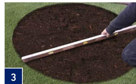
Create an even, level area using your shovel to remove any high spots. Ensure that the surface area inside the circle is level using a standard household level.
