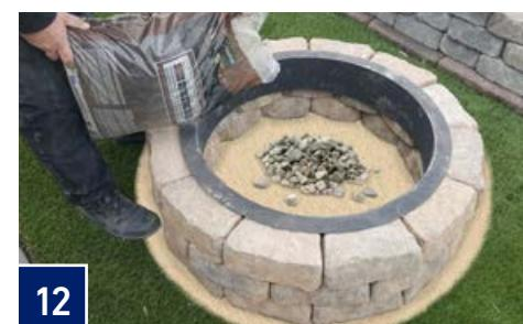
After the concrete adhesive has dried, fill the bottom of the fire pit with gravel/lava rock, leveling the material as you fill. Gravel/lava rock should fill up to the bottom edge of the steel fire ring.
