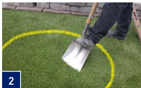
Using a shovel, remove all sod, dirt, roots and any other organic material, digging to an even depth of 2" within the area of the circle.
