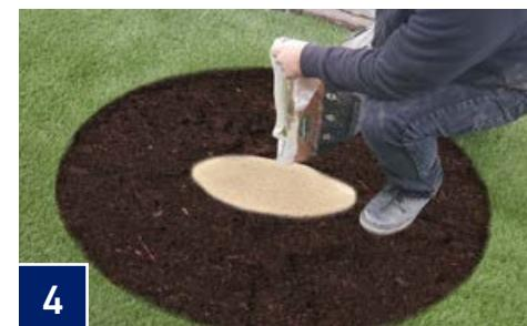
Pour 1 1/2" to 2" of paver base/coarse sand inside the excavated area, ensuring that the height of the sand is even and level. Mist the sand with water and use a hand tamper to evenly compact the entire area inside the circle. Pour an additional 1/2" to 1" of paver base/sand into circular area and level. Do not compact.
