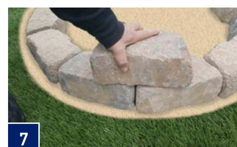
This step is called "dry fitting" to ensure positioning of block before adhering in place in step 8. When laying the second course of blocks, be sure to follow a "one over two" pattern, aligning middle of the each block over the joint made between two blocks under it. Ensure blocks are level front to back and side to side as you complete ring of second course.
