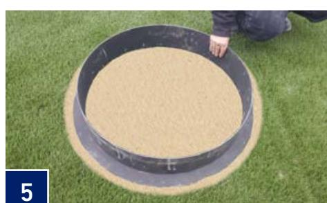
Carefully place steel fire ring, flange side down into the paver base/sand creating an indentation. Carefully lift the fire ring straight up, trying to disturb as little paver base/sand as possible. This step will create a circular mark, or guide for you to begin placing the block for your Firepit Kit.
