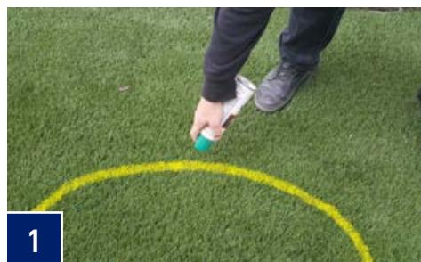
When installing Firepit Kit on a grass area or lawn, mark out a 49" (125cm) diameter circle using marking paint and proceed to Step 2. If installing on a suitable patio area, use chalk rather than paint to draw a 49" (125cm) diameter circle and proceed to Step 5.
