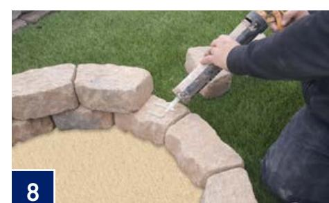
Lift one block at a time from its position on the second course and apply two thick beads of concrete adhesive, near the center of stone and 2" inches apart. The beads should run parallel with the wall face (end to end not front to back). Replace stone in original position pressing down firmly while twisting slightly.
