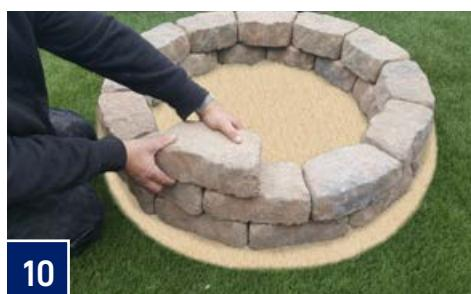
Dry fit third course of blocks with the joints at the ends aligning with the joints on first course. Apply adhesive as previously instructed in Step 8. After all blocks are in place, and while adhesive is still fresh, slide the steel fire ring into the center of the project. Block may move slightly or need to be slid outward to allow fire ring to drop into place.
