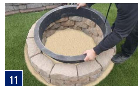
The outside lip of the steel fire ring will rest on the inside edge of the wall block. Ensure that the ring is completely embedded and the lip of the ring is in contact with top surface of block around third course. Re-align block if necessary by tapping them back against steel insert and evening out any large gaps between block ends.
