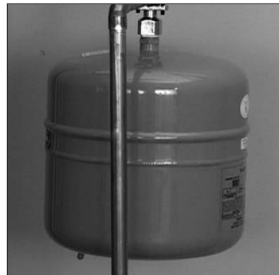
Figure 55. The Thermal Expansion Tank should be pressurized with air to match the home's incoming water pressure.
