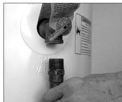
Figure 20. Removing the T&P Relief Valve discharge pipe.
