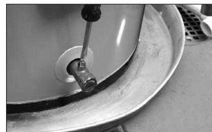
Figure 19. Draining the old water heater.
