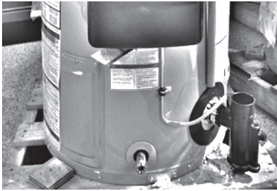
Figure 26. Condensate/Exhaust Tee Installation
