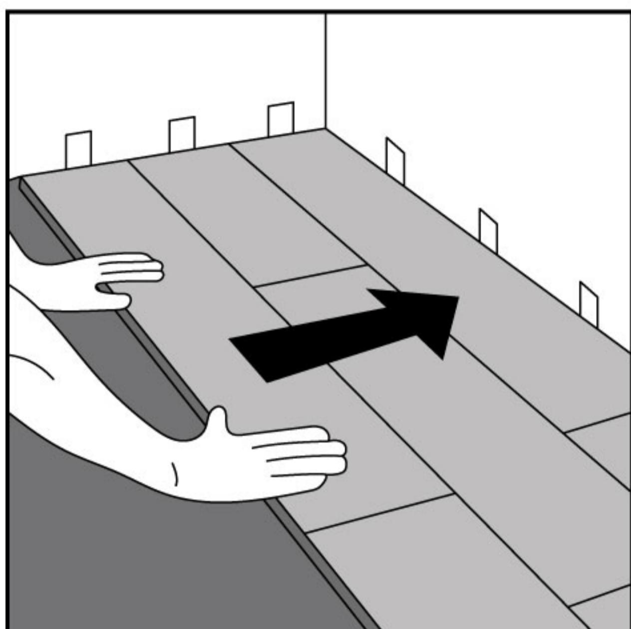
After 2-3 rows. Adjust the distance to the front wall by leaving an expansion gap of 1/4". Always ensure that the end joints are staggered at least 8", both when in the same row as when from one row to the next one.
