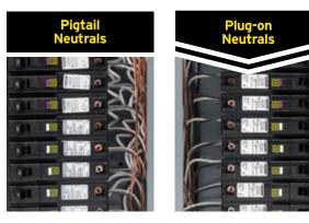
Plug-on Neutral load centers and Combination Arc Fault and Dual Function breakers from Square D simplify installation, saving you time, labor and cost.
