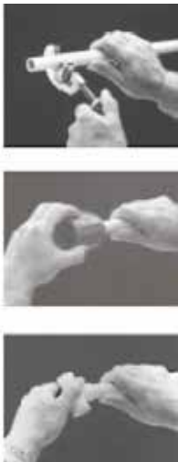
Check dry fit Photos A-B-C
