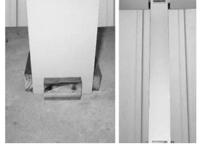
3) If desired, optional blocking (not provided) may be installed around post to center wrap. This is especially helpful when wrapping round or odd sized supports.
