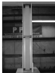
8) Place the partially assembled (three panels) column around post and blocking.
