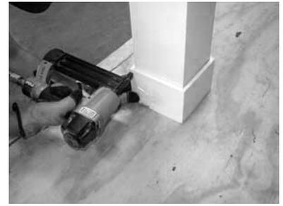
12) Fasten joints on base with pin-nails.
