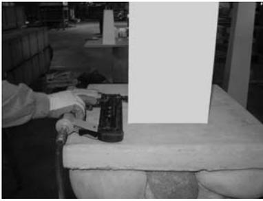
10) Screw or nail column to blocking **ONLY ON THE BOTTOM**. Do not attach at center or top (to allow for expansion).
