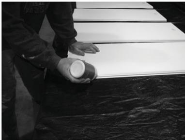
3) Apply polyurethane glue to both edges of ONE PANEL only.
