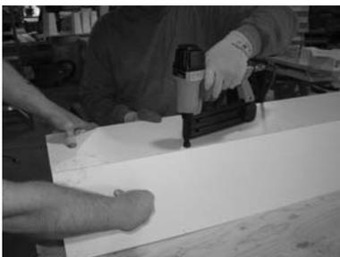
7) Using finish nails, assemble three panels together. Observe E-Z Lock diagram on reverse to determine correct nail placement.
