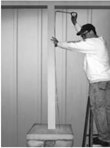
1) Measure overall opening height from floor to beam or soffit (must have structural pressure-treated post or lally column for load support.)
