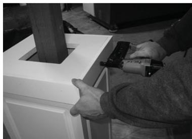
10) Apply glue to backs and mitered edges of cap moldings, then assemble to shaft below top platform with pin-nails. (Mouldings, panels, trim, and top platforms may vary from photos depending on product styles.)
