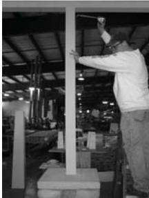
1) Measure overall opening from floor to beam or soffit (must have structural pressure-treated post or lally column for load support.)
