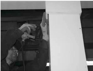
16) Option 2: Leave 1/4" expansion room above cap, and pin-nail the cap to the column. Be sure the pin-nails **DO NOT** reach the blocking inside!\*
