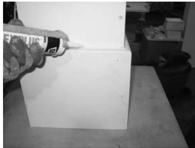
17) Caulk edges of base, cap, and nail holes.
