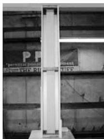
8) Place the partially assembled (three panels) column around post .
