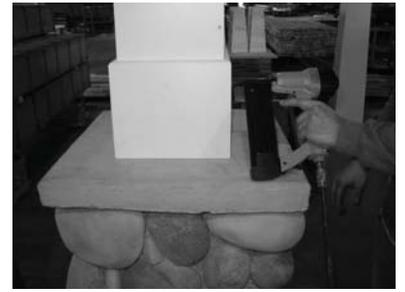
12) Fasten joints on base with pin-nails.
