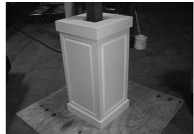
11) Caulk all seams, fill all nail holes, and clean surfaces with cleaner recommended by paint manufacturer. Finish with two coats of acrylic latex paint.
