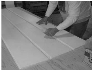
5) Lay 3 panels flat and apply adhesive to center joints. (Polyurethane glue is recommended. Follow manufacturer's instructions.)
