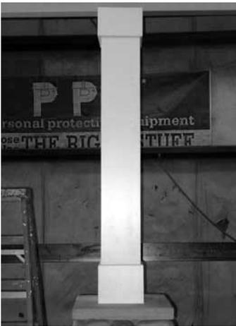
16) Clean surface of column with cleaner recommended by the paint manufacturer. (Do not use solvents). Allow to dry completely, then paint with 2 coats of acrylic latex paint. **Warning: using dark colors might cause excessive thermal expansion.**
