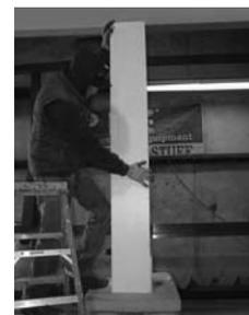
9) Apply adhesive to fourth panel and attach to shaft using E-Z Lock joints. Pin-nail in place.
