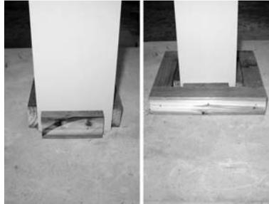
2) Install blocking around load bearing post (use pressure treated lumber.) Final width of blocking must be same width as inside of column.
