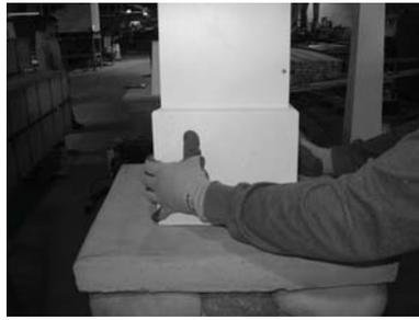
11) Apply adhesive to mitered edges of base moulding (standard base is 9 1/4" tall) and assemble around bottom of column shaft.
