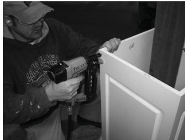
7) Glue and attach final panel. For use as a newel, additional blocking should be added between panels and post (post would be cut off at height of shaft.)
