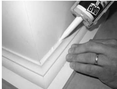
17) Caulk using latex caulking compound to fill any gaps and nail or screw holes.
