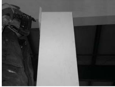
14) There are **TWO** methods of attaching the cap. First, apply adhesive to mitered edges of cap moulding (7 1/4" tall) and assemble around shaft and pin-nail joints.
