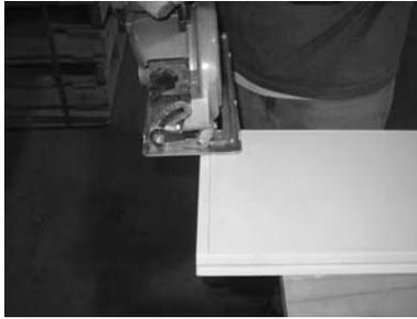
2) PVC expands and contracts with temperature changes. Trim shaft pieces to 1/2" shorter than opening height (from step 1) to allow for product expansion.
