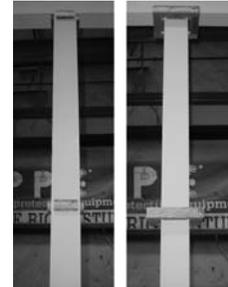
3) Install blocking around center and top of post to match step 2 (center blocking is optional.) Blocking may be attached to deck/soffit instead of post if necessary.
