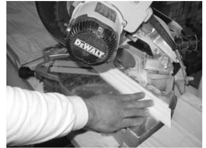
15) If base trim moldings are too long, use miter saw to cut base trim pieces to fit around bottom of column.\*\*
