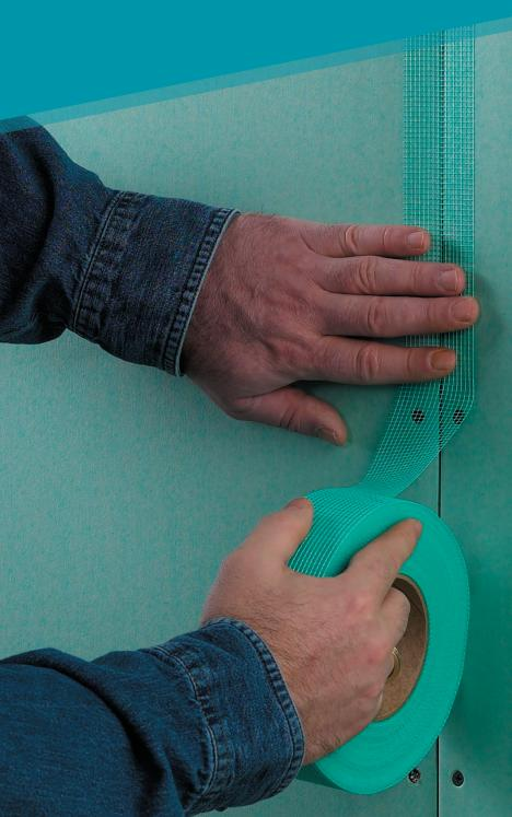
Designed specifically for use with mold resistant board
