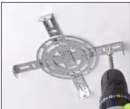
3. Secure each arm of the hanger by fixing them to the ceiling with the help of the wood screws.
