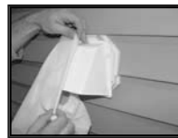
Position LintCatcher over the vent
