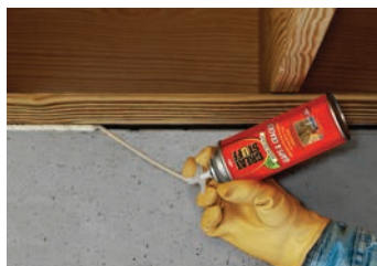
Rim joist/Sill plate
