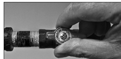
Figure 51 - Gas valve in "on" position.
