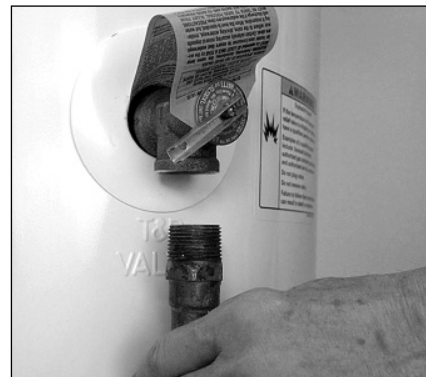
Figure 21 - Removing the T&P Relief Valve discharge pipe.
