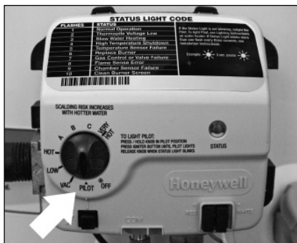
Figure 34 - Gas control/valve.
