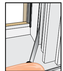
Pry off Monumental Double-Hung jamb liner
