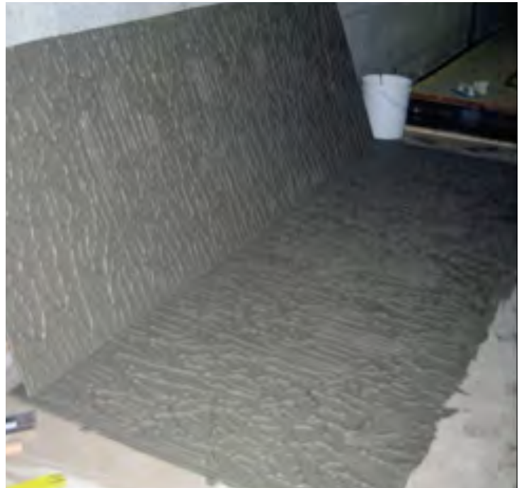
Example of proper full mortar coverage
