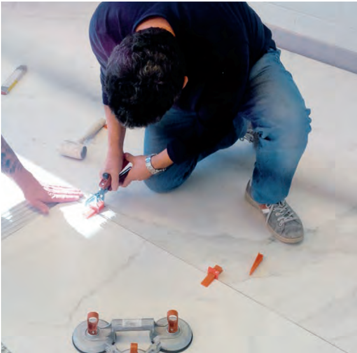
Self-leveling system being used for floor installation
